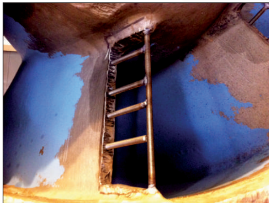
A threaded rod "skeleton" was installed by tack welding to the already cut vanes.
